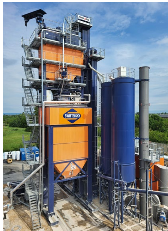
Asphalt mixing plant, Székesfehérvár, Hungary
