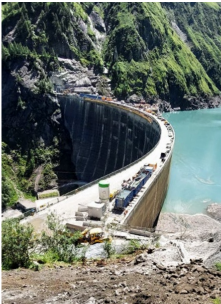
Kühtai, Austria Raising the Limberg dam, Kaprun, Austria Rathaus/Frankhplatz metro station, Vienna, Austria
