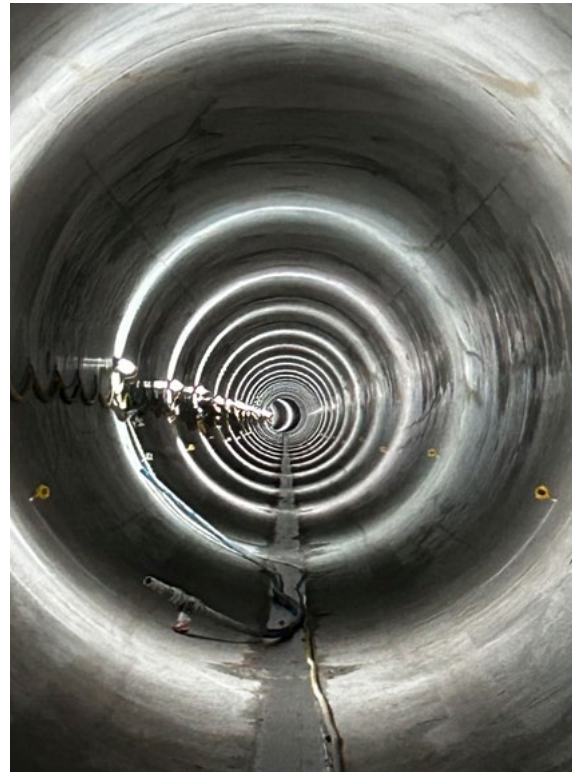
Tauernbach-Gruben power plant, Matrei in Osttirol, Austria
